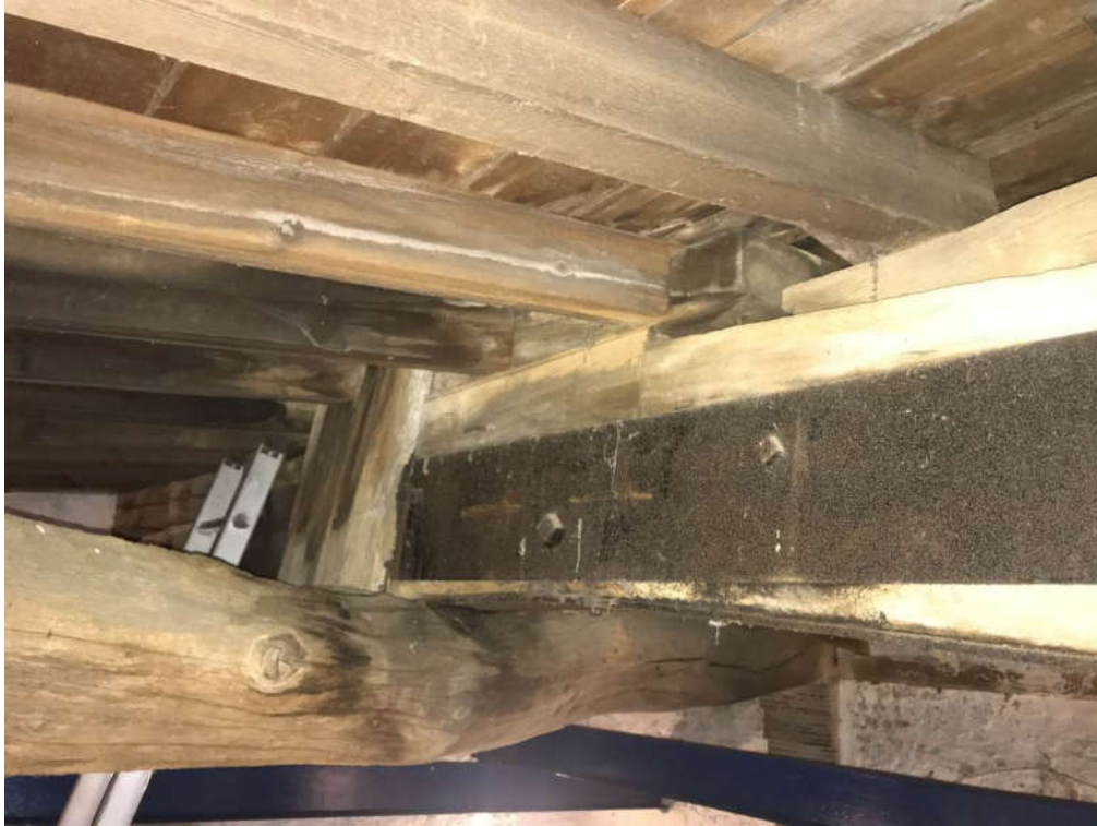
Photograph 7 – Weathervane post fixed to side of ridge beam
