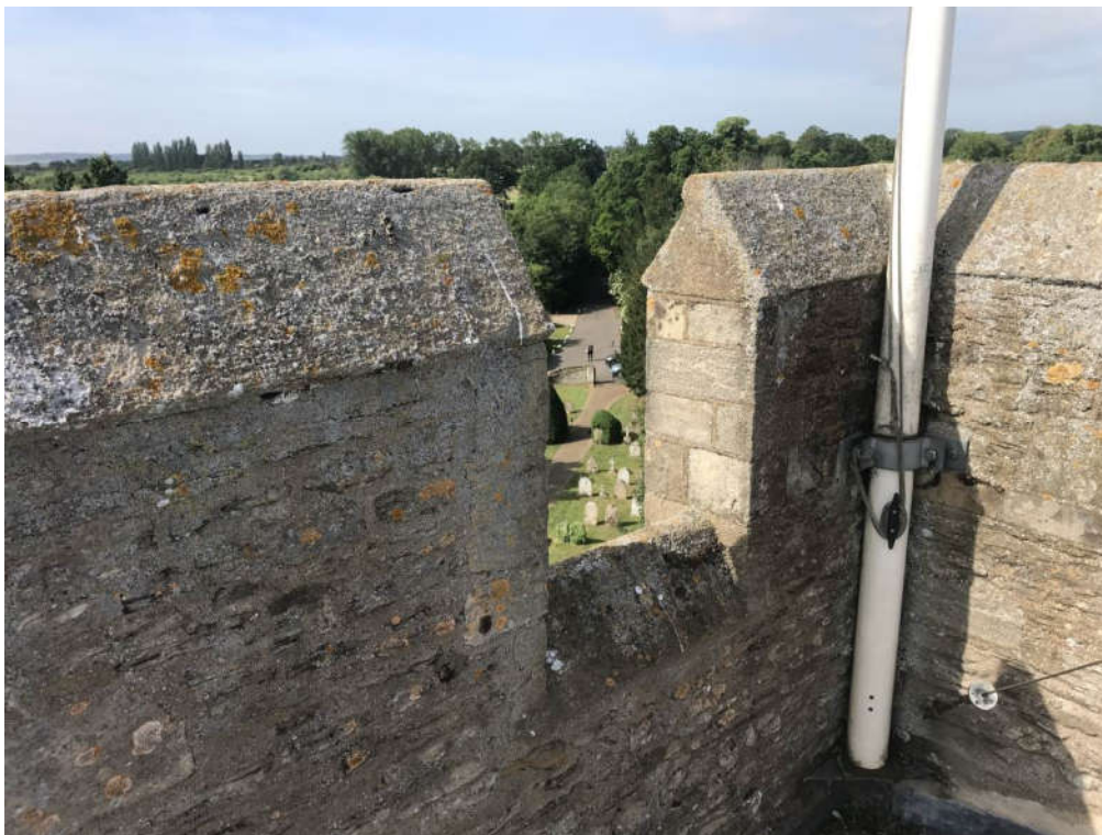
Photograph 12 – Flagpole fixed to parapet wall
