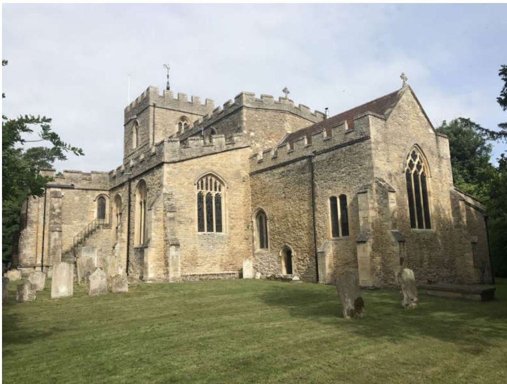
Photograph 2 – South East corner of church
