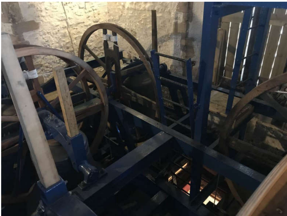
Photograph 6 – 'Modern' steelwork to support bells
