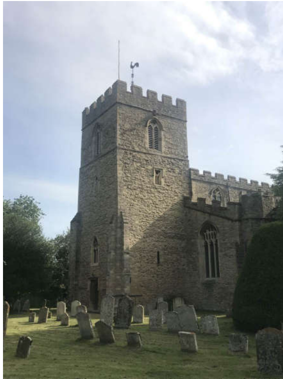
Photograph 1 – South West corner of tower
