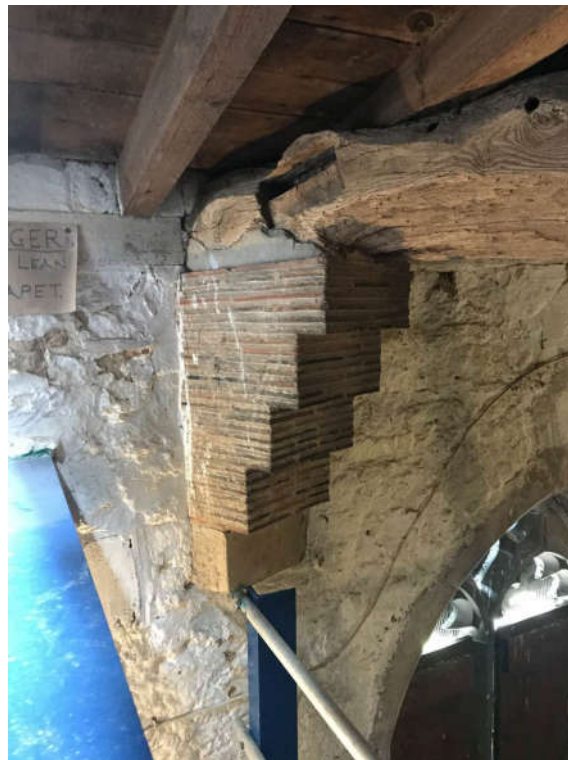
Photograph 8 – Principal support beam bearing on corbelled tile construction
