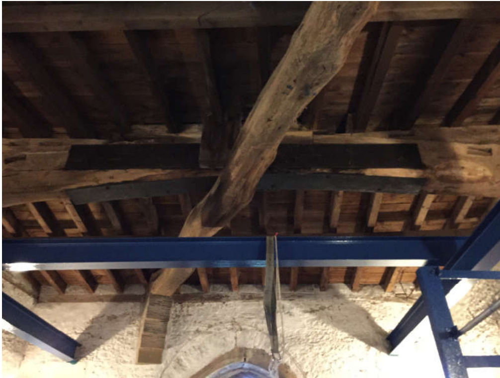
Photograph 5 – Principal support beam supporting strengthened ridge beam
