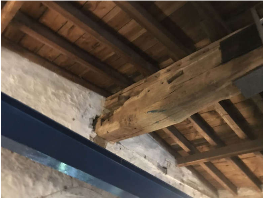
Photograph 9 – Ridge beam support
