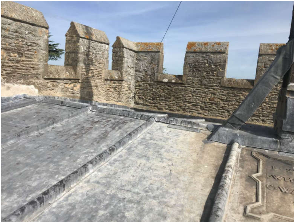
Photograph 3 – Tower roof finished in lead
